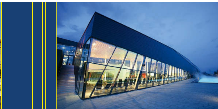
The Fohnsdorf Aqualux Spa in Styria has a gross floor space of 9,000 m 2 and a pool and spa area of 900 m 2 . It was built in just 14 months.
