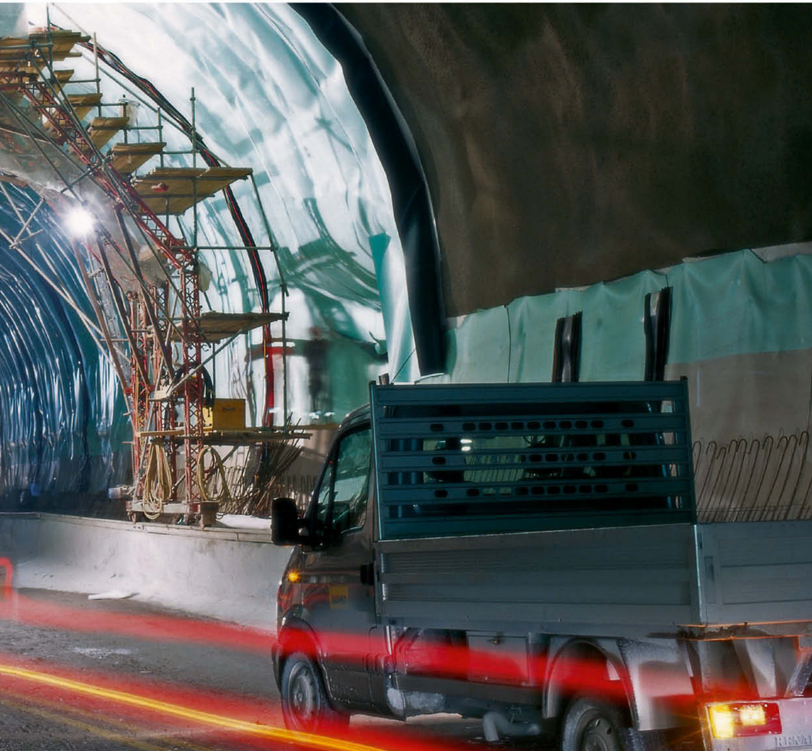
Brixlegg tunnel, Tyrol
