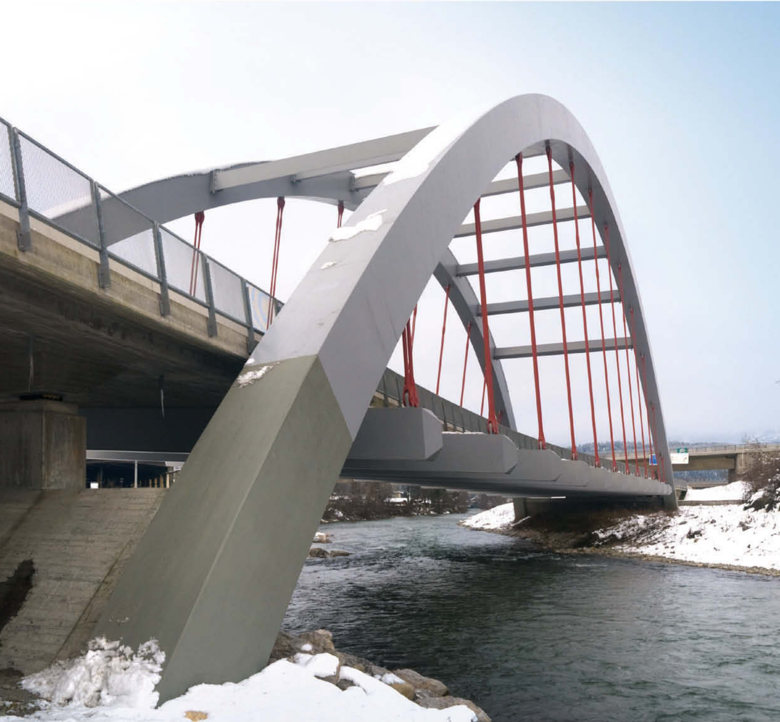
Wörgl-Bruckhäusl By-pass, project unit 3, Tyrol
