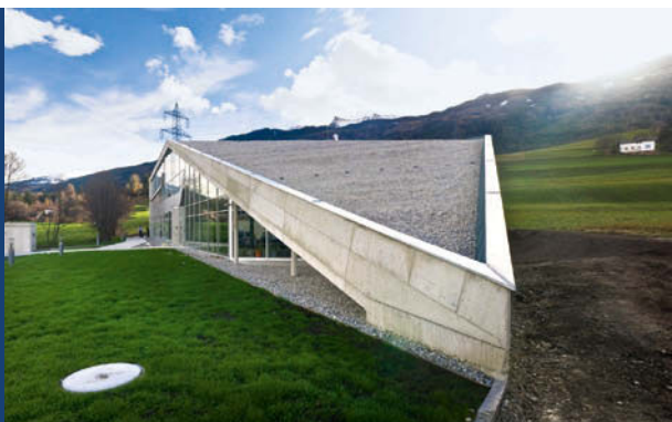
The Aldrans-Lans-Sistrans Entrepreneur Centre lies south east of Innsbruck. Here top residential comfort sits happily alongside commercial space ( www.unternehmerzentrum.at ).
