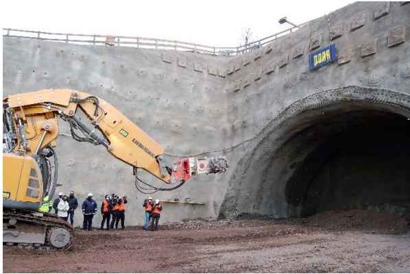
Tunnel boring for TS-26 on the S3 route ©PORR
