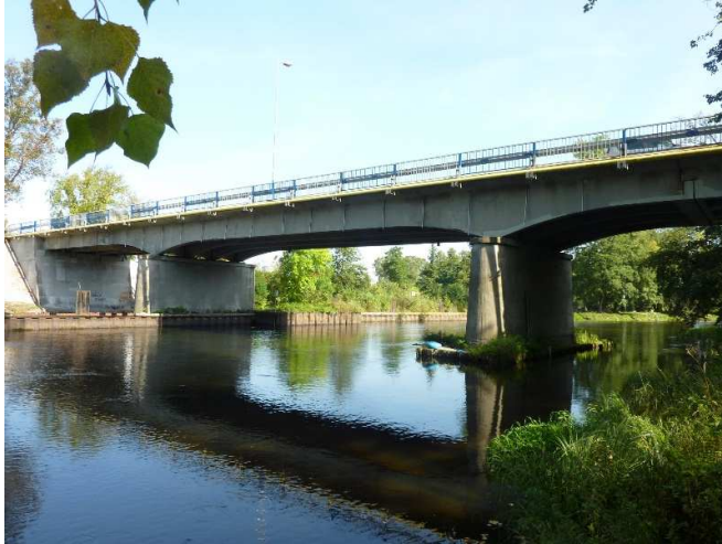
Bridge over the Gwda River in Ujście © GDDKiA
